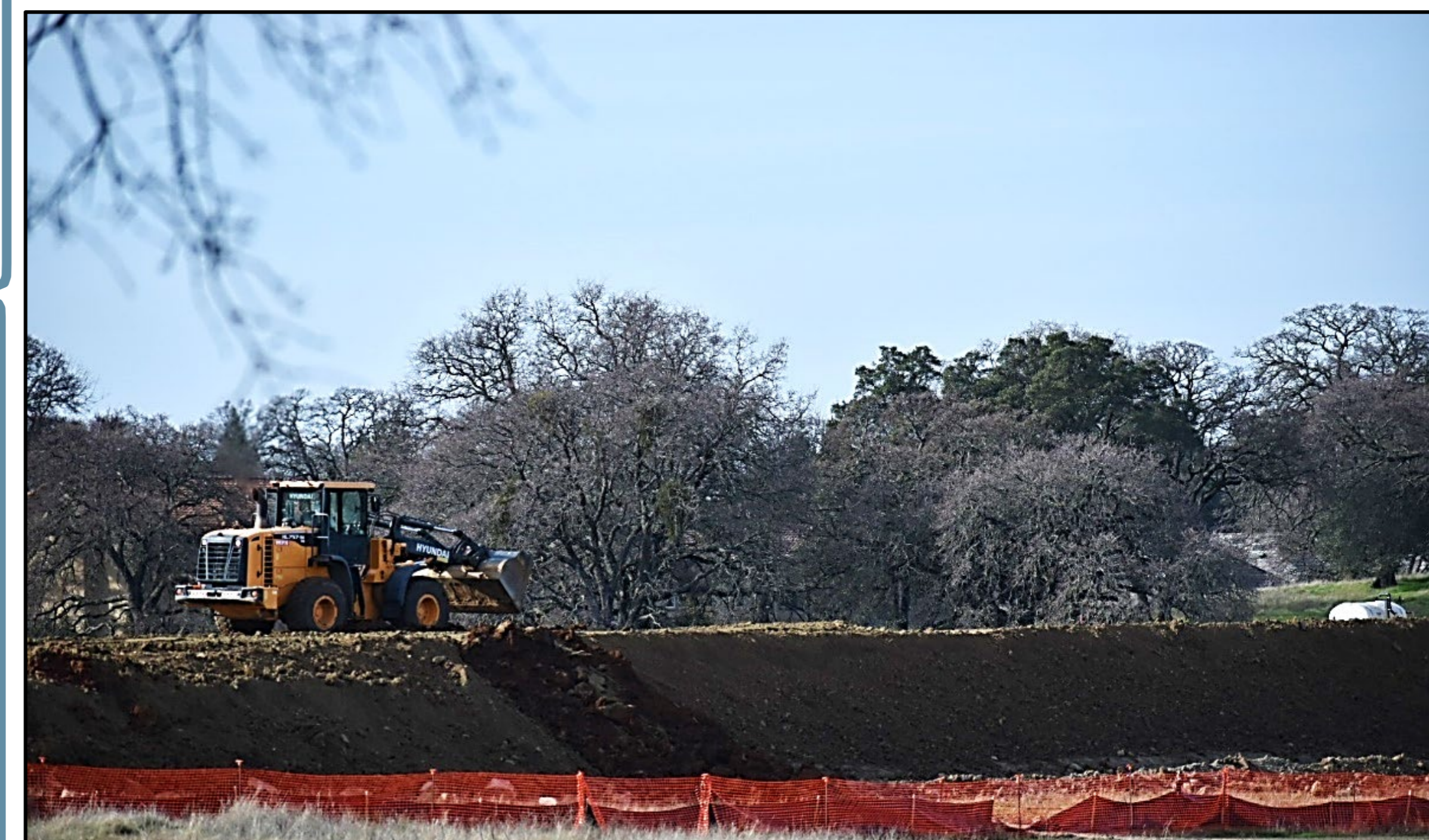
Construction at Dike 8
